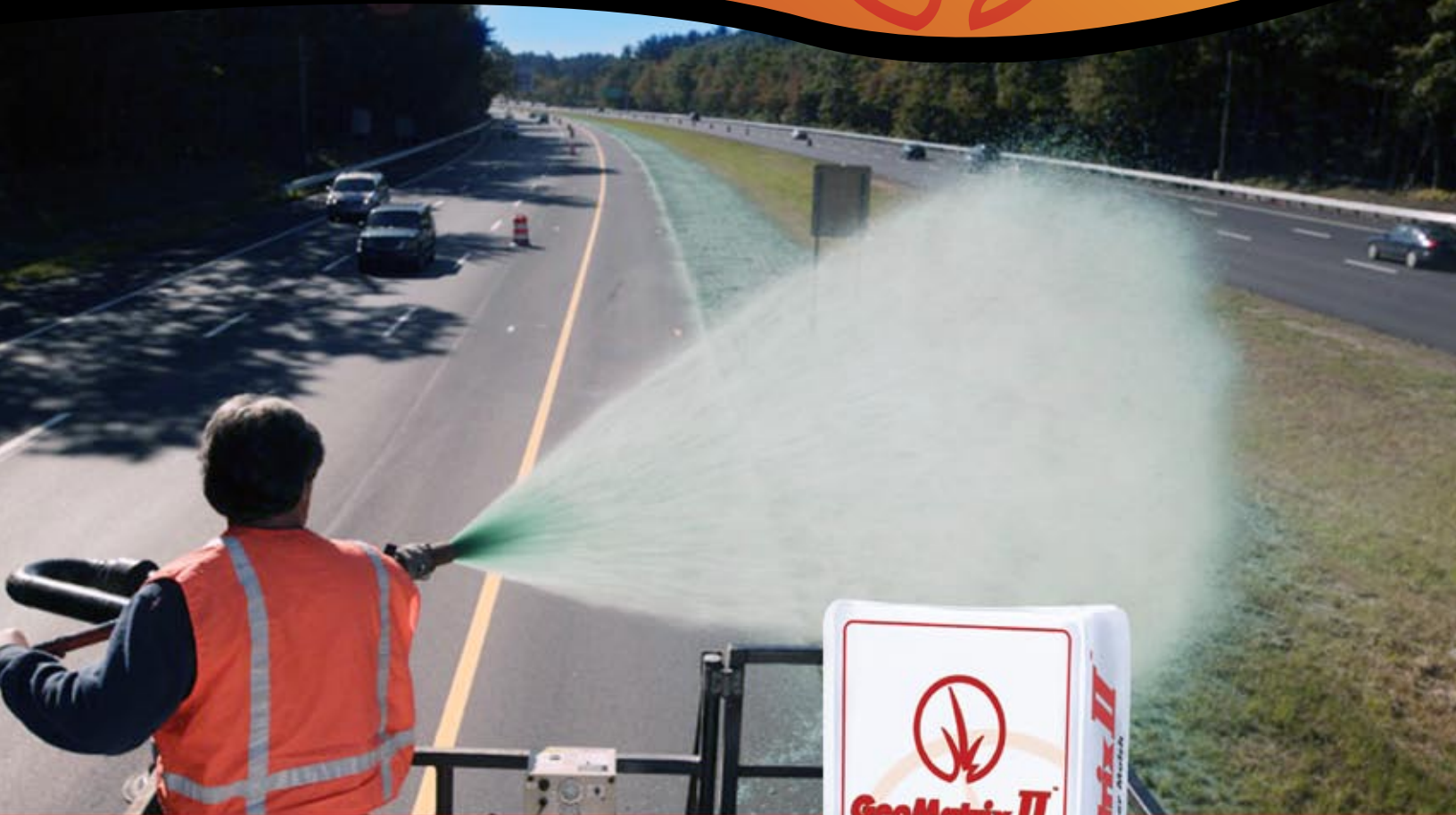
GeoMatrix II being applied from tower
